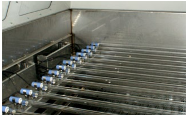
Irradiation with ultraviolet light neutralizes odours and ensures good air.
